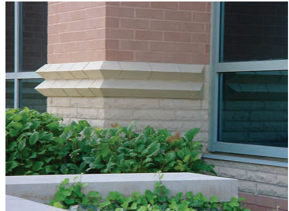
Projected Stretcher and Projected Stretcher Corner
