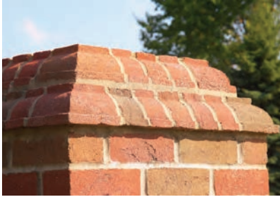
Watertable Rowlock External Corner & Watertable Rowlock
